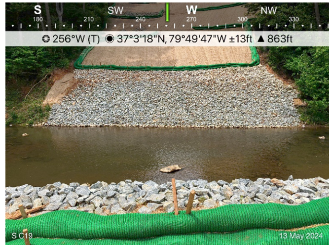
Figure 2: Designated crossing S-C19, ESC and permanent measures in place.
