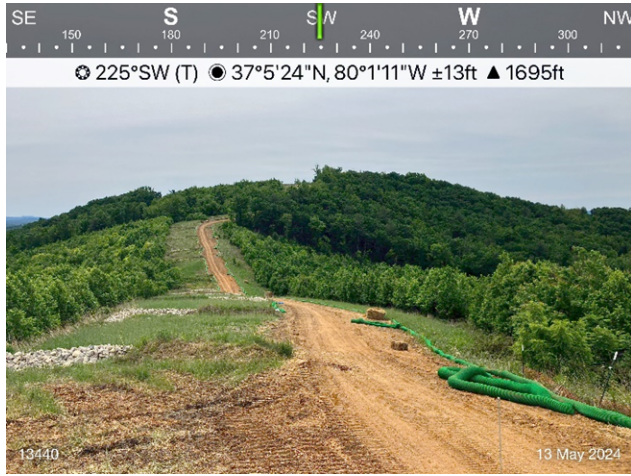
Figure 1: Sta 13340, perimeter controls in place.
