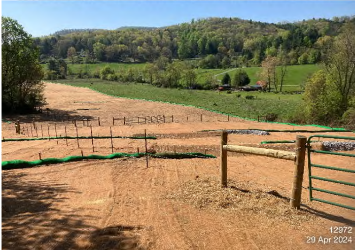
Figure 3: STA 12991+00 – Controls in place and functioning properly.
