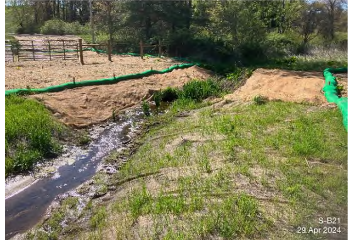
Figure 4: Stream S-B22 – Controls in place and functioning properly.
