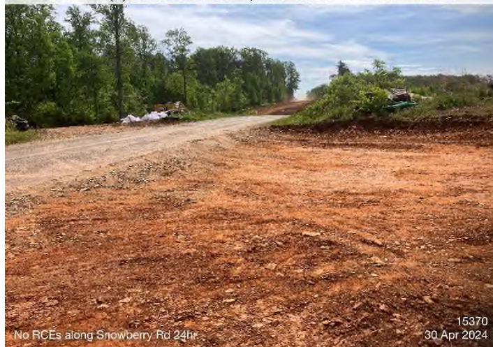
Figure 3: STA 15435+00 – Sediment discharged off ROW.
