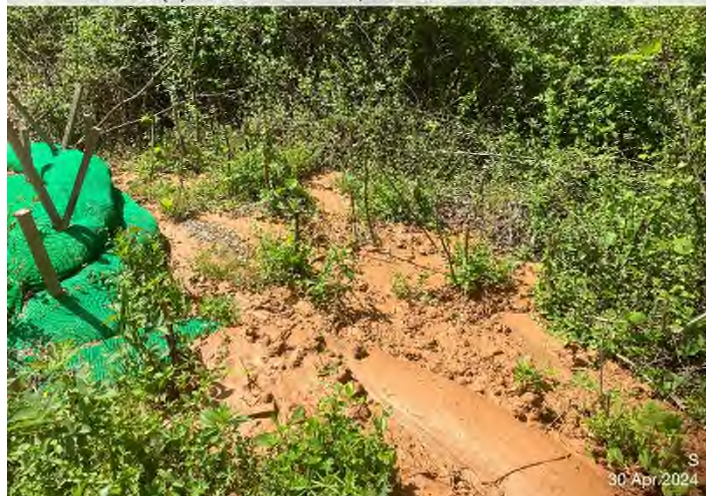
Figure 3: STA 15435+00 – Sediment discharged off ROW.
