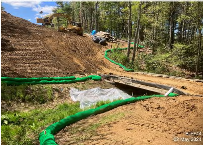
Figure 3: Stream S-EF44 – Controls in place and functioning properly.
