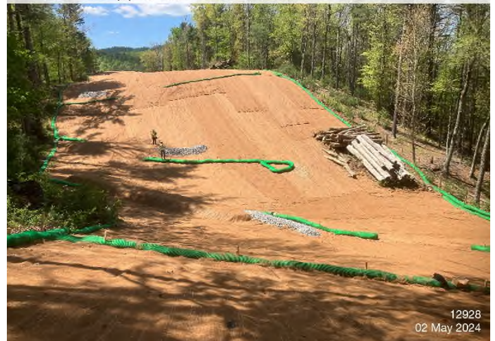
Figure 4: STA 12928+00 – Controls in place and functioning properly.
