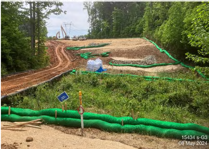
Figure 3: Stream S-G3 – Controls in place and functioning properly.
