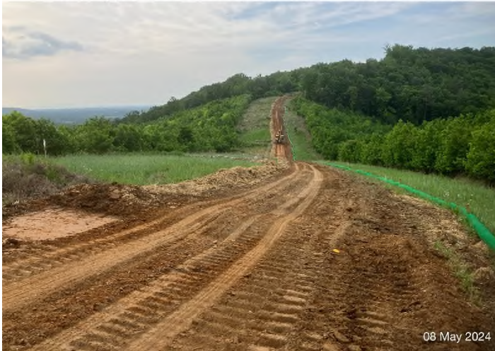
Figure 3: Stream S-G3 – Controls in place and functioning properly.
