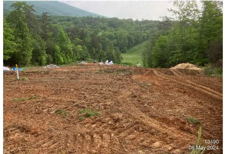
Figure 4: STA 14230+00 – Controls in place and functioning properly.
