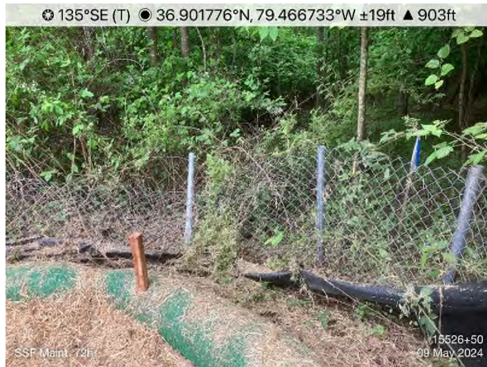
Figure 23: STA 15616+00 – Waterbar end-treatment improper installation. Install per specification.
