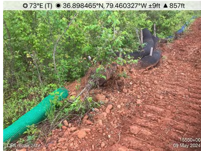
Figure 20: STA 15548 to STA 15550+00 – CFS repair needed.
