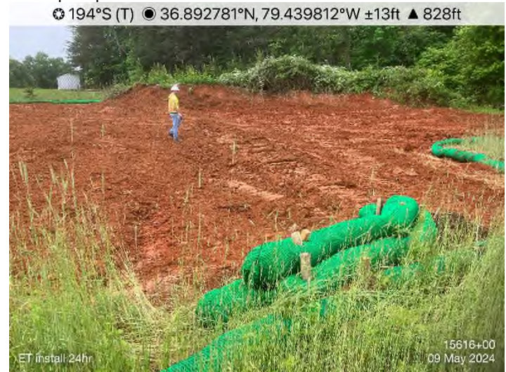
Figure 24: STA 15616+00 – Waterbar improper installation. Install per specification.
