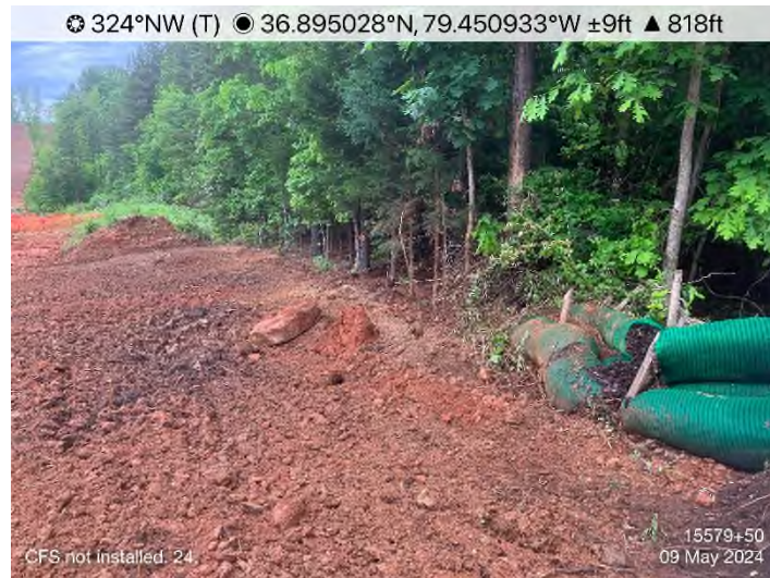
Figure 3: STA 15579+50 – CFS not installed, CFS repair needed.
