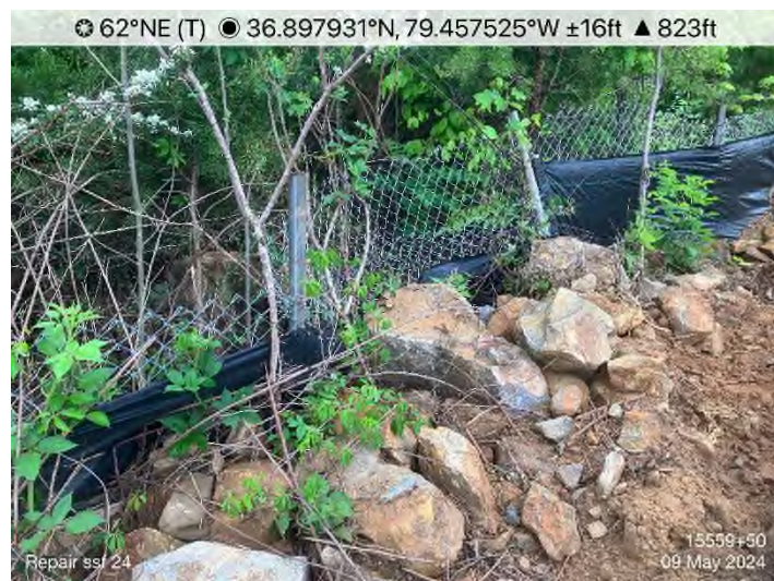
Figure 19: STA 15552+00 – Sediment off ROW from grading activities. Retrieve and stabilize as needed.
