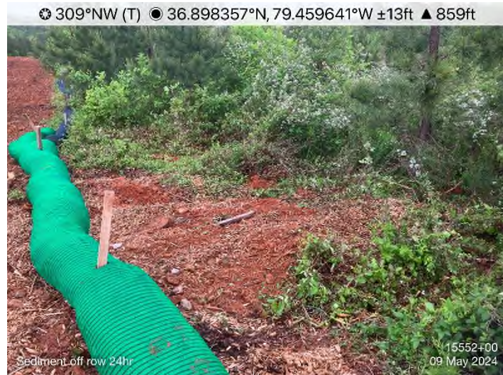
Figure 19: STA 15552+00 – Sediment off ROW from grading activities. Retrieve and stabilize as needed.
