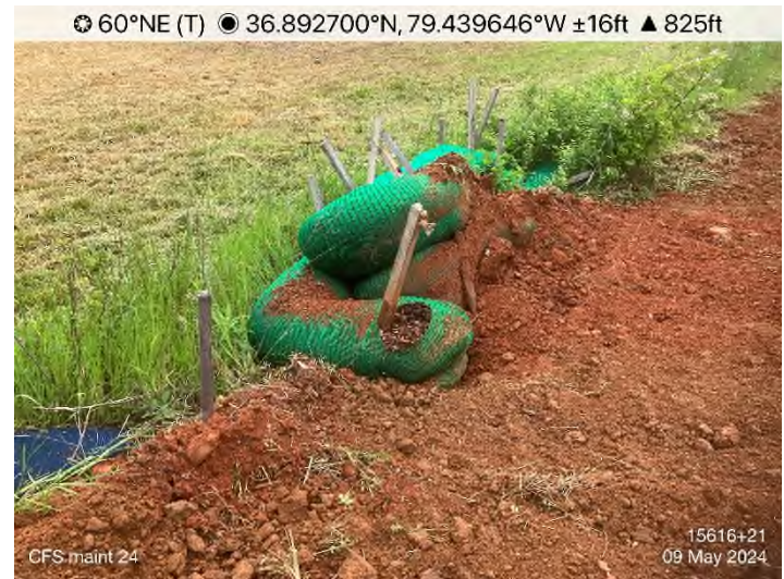
Figure 24: STA 15616+00 – Waterbar improper installation. Install per specification.
