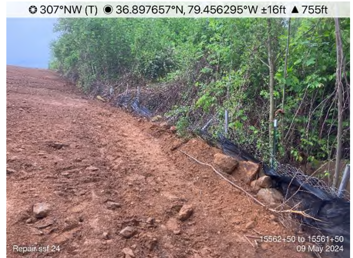
Figure 16: STA 15561+50 to STA 15562+50 – SSF repair needed.
