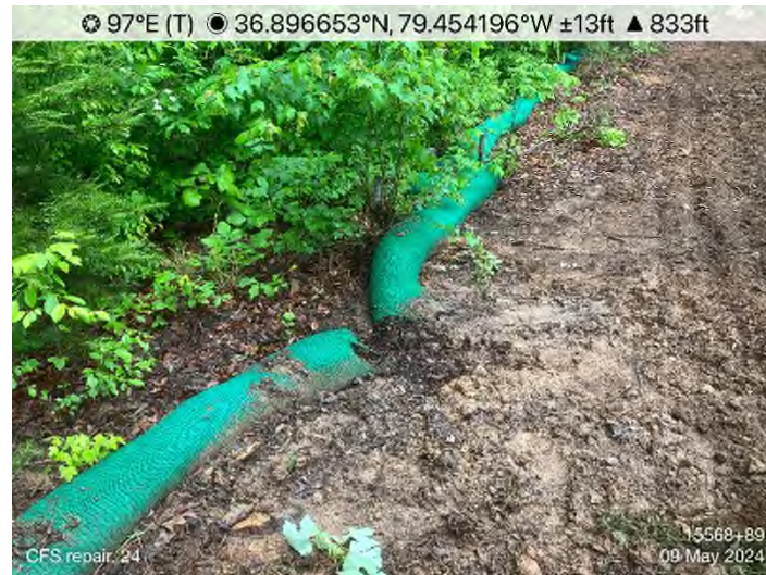
Figure 8: STA 15568+90 – CFS repair needed.
