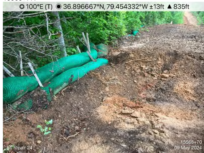
Figure 10: STA 15568+70 – Waterbar end-treatment not installed/repared by the end of the day causing SOR at STA 15568+77.
