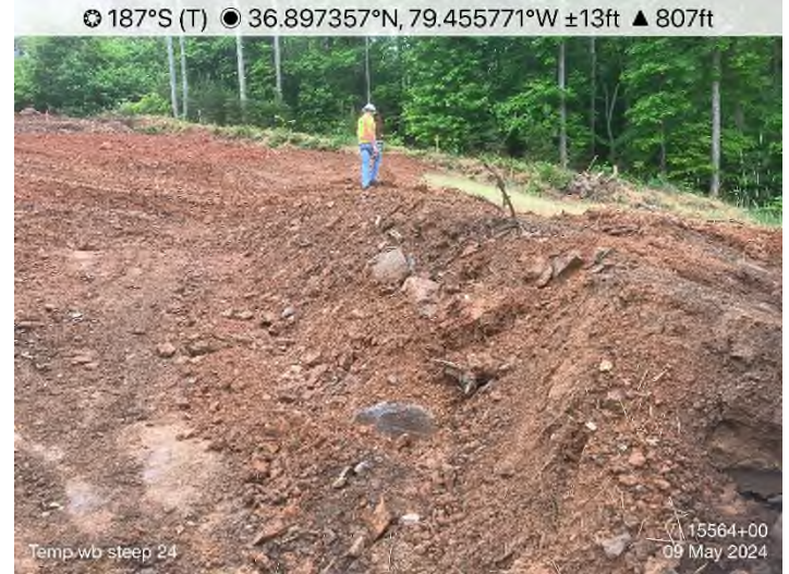
Figure 14: STA 15564+00 – Temp. WB improper install, too steep, not compacted. Install per specification.
