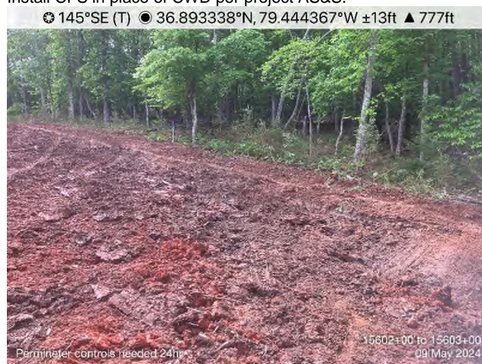
Figure 30: STA 15602+00 to 15603+00 – Controls not installed. Install CFS in place of CWD per project AS&S.
