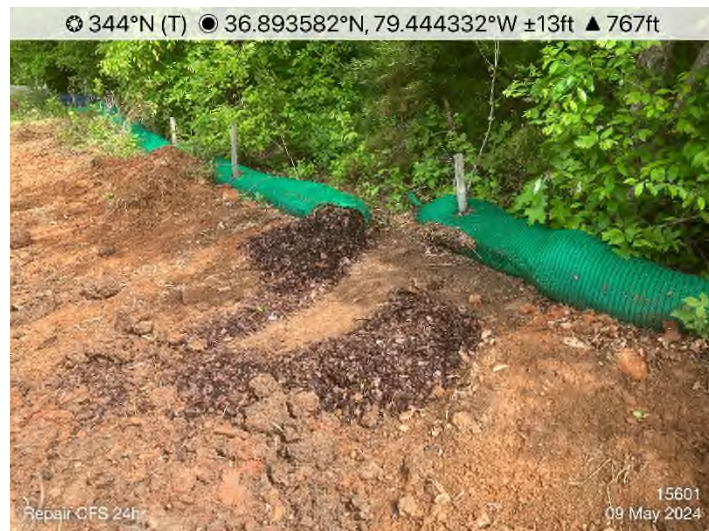
Figure 31: STA 15601+00 – CFS repair needed.
