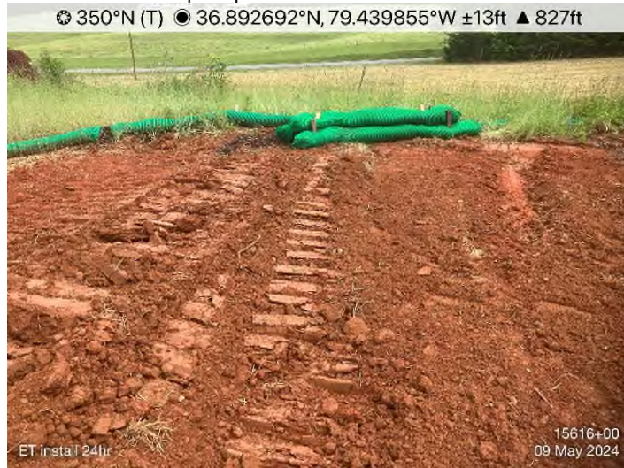
Figure 23: STA 15616+00 – Waterbar end-treatment improper installation. Install per specification.
