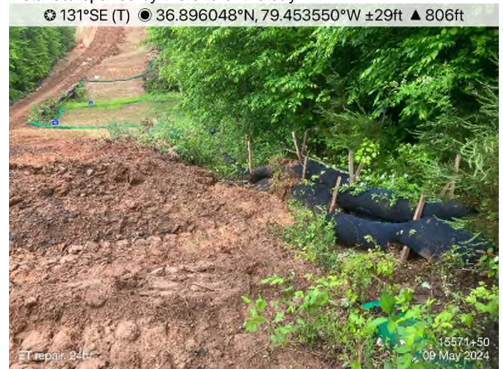
Figure 4: STA 15571+50 – Waterbar end-treatment not installed/repared by the end of the day.
