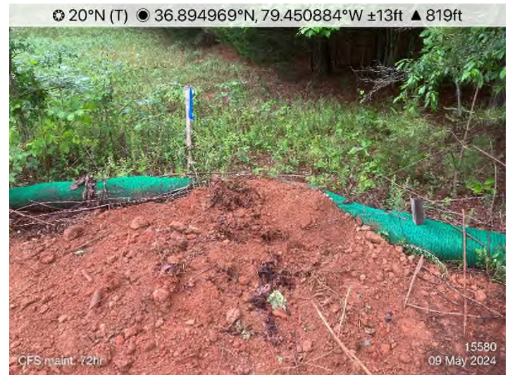
Figure 4: STA 15571+50 – Waterbar end-treatment not installed/repared by the end of the day.
