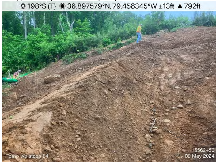
Figure 15: STA 15562+50 – Temp. WB improper install, too steep, not compacted. Install per specification.
