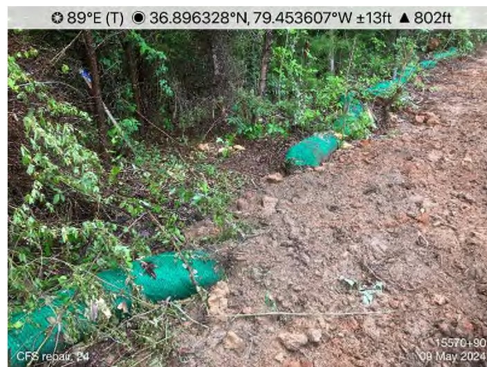
Figure 8: STA 15568+90 – CFS repair needed.
