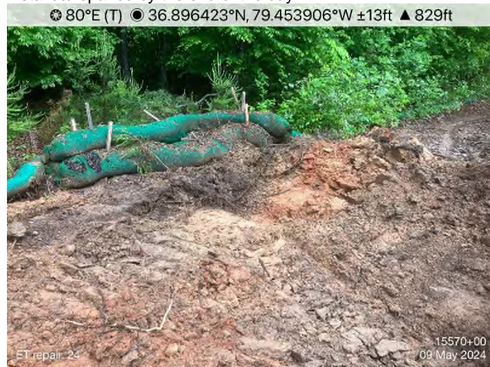
Figure 7: STA 15570+00 – Waterbar end-treatment not installed/repared by the end of the day.
