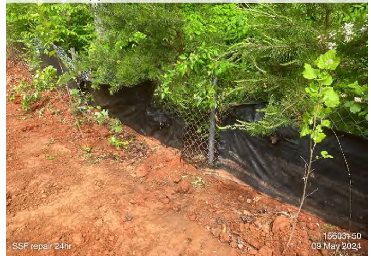
Figure 28: STA 15603+50 – SSF repair needed.
