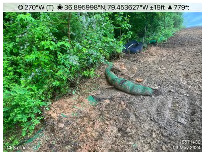
Figure 7: STA 15570+00 – Waterbar end-treatment not installed/repared by the end of the day.
