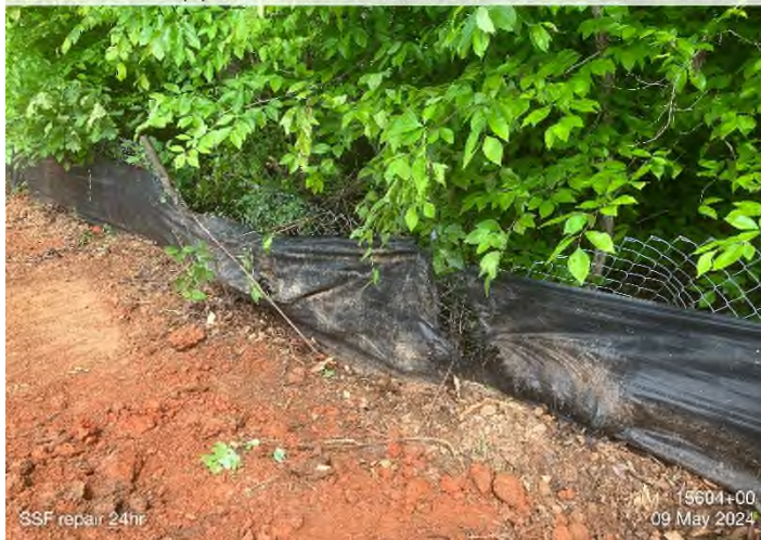
Figure 27: STA 15604+00 – SSF repair needed.
