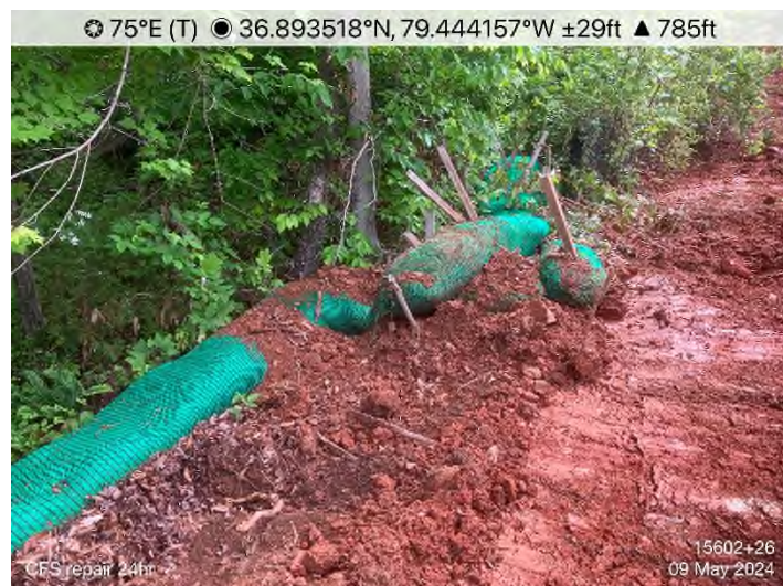
Figure 31: STA 15601+00 – CFS repair needed.
