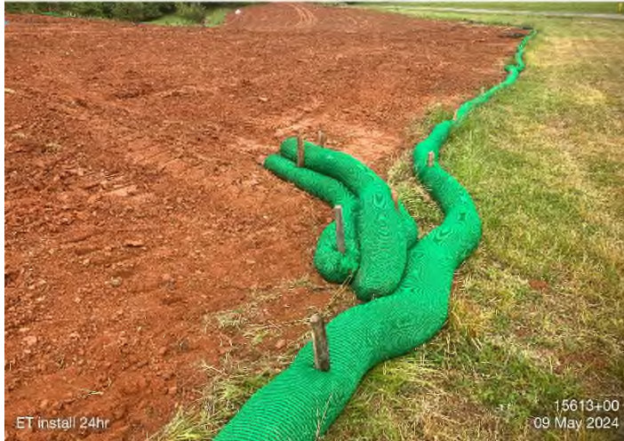
Figure 27: STA 15604+00 – SSF repair needed.
