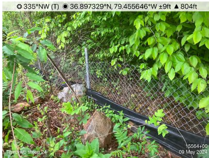
Figure 15: STA 15562+50 – Temp. WB improper install, too steep, not compacted. Install per specification.
