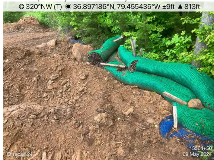
Figure 12: STA 15564+50 – Waterbar end-treatment not installed/repared by the end of the day.
