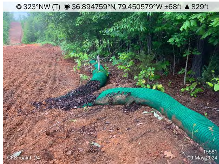
Figure 3: STA 15579+50 – CFS not installed, CFS repair needed.
