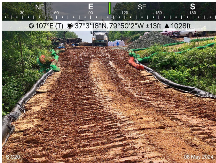
Figure 3: Designated crossing S-C20, ESC is in place for active construction.
