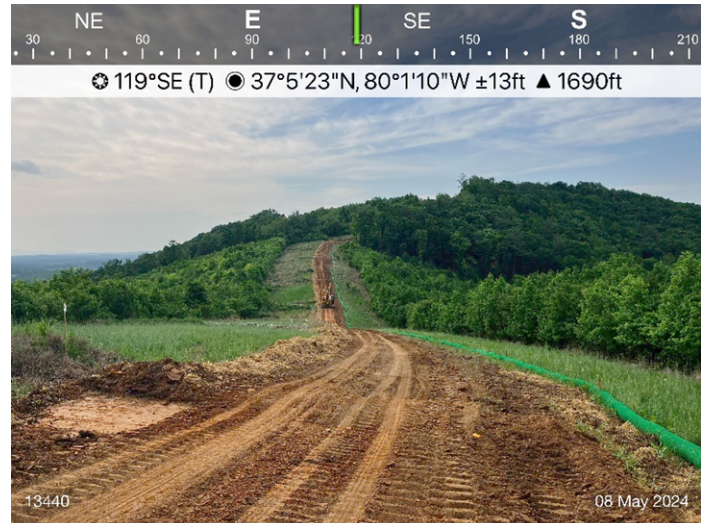
Figure 4: Sta 13440, ESC is in place.
