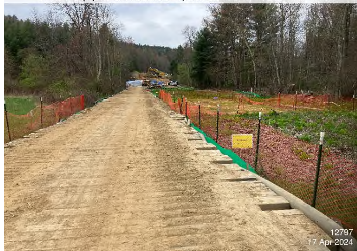
Figure 3: Wetland W-IJ95 – Controls in place and functioning properly.
