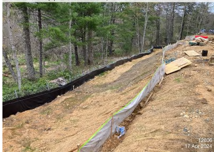
Figure 4: STA 12806+00 – Controls in place and functioning properly.
