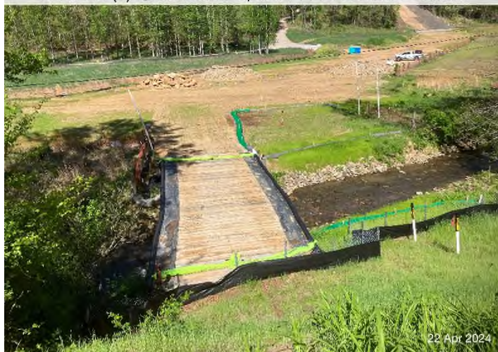
Figure 4: Stream S-D8 – Controls in place and functioning properly.
