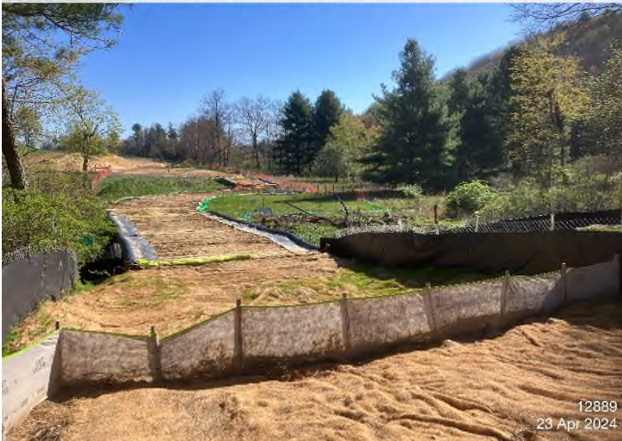
Figure 3: STA 12889+00 – Controls in place and functioning properly.
