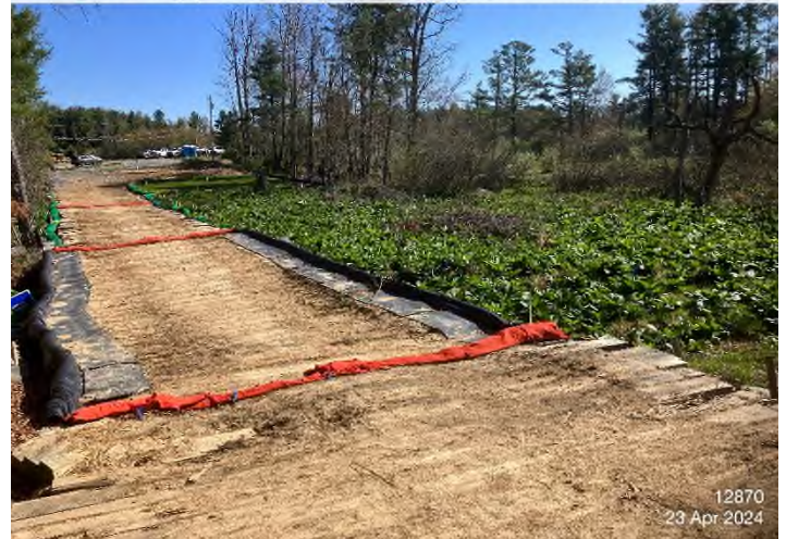
Figure 4: STA 12870+00 – Controls in place and functioning properly.
