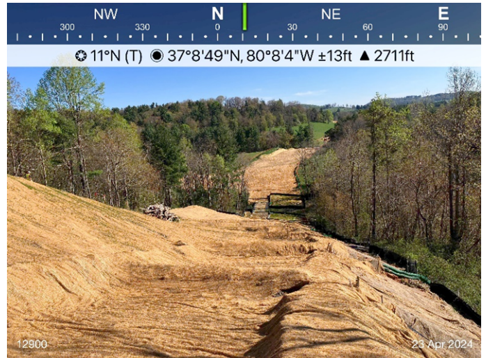
Figure 2: Sta 12900, ESC's devices in place.
