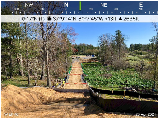
Figure 3: Designated crossing W-EF46, ESC's devices in place.
