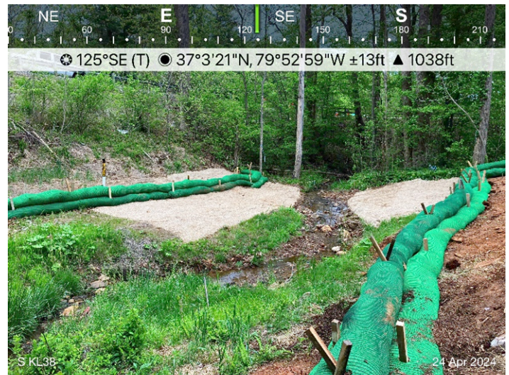
Figure 4: Designated crossing S-KL38, ESC is in place.
