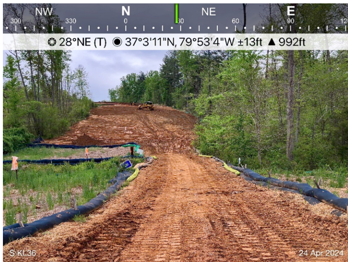
Figure 3: Designated crossing S-KL36, ESC is in place.
