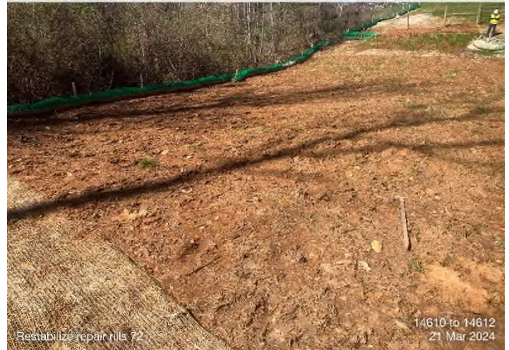
Figure 4: STA 14610+00 to 14612+00 – Repair rilling and restabilize denuded areas.
