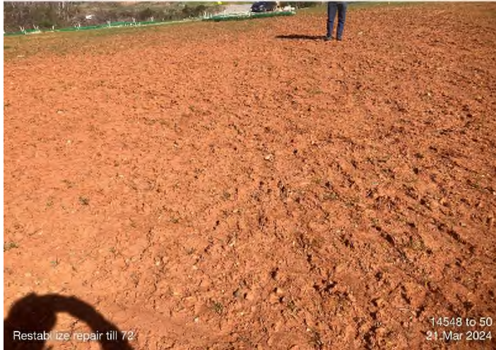
Figure 3: STA 14568+50 to 14569+50 – Repair rilling and restabilize denuded areas.
