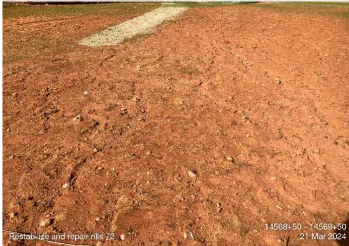
Figure 3: STA 14568+50 to 14569+50 – Repair rilling and restabilize denuded areas.
