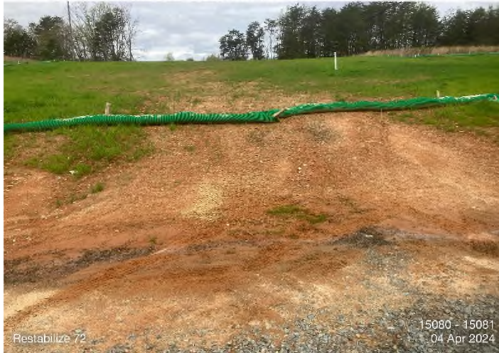
Figure 1: STA 15080+00 to 15081+00 – Repair rilling and restabilize denuded areas.
