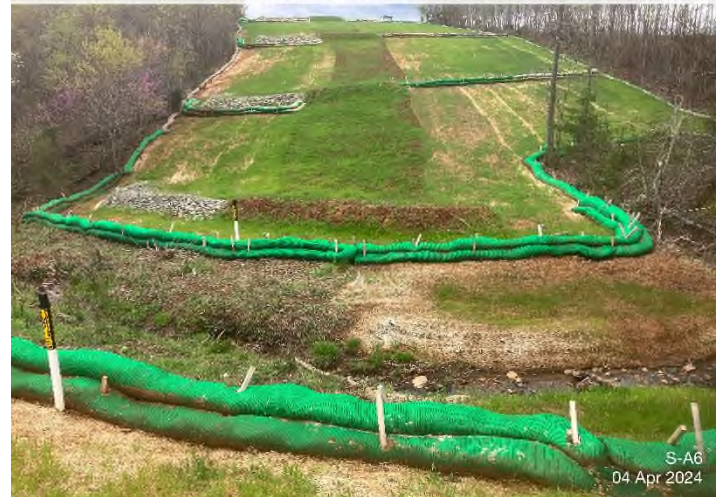
Figure 4: Stream S-A6 – Controls installed and functioning properly.
