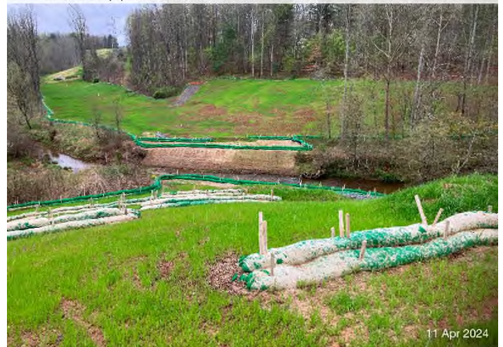
Figure 4: STA 13831+00 – Controls in place and functioning properly.
