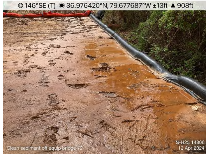
Figure 5: STA 14806+00 – Remove sediment accumulation from equipment bridge crossing over Stream S-H23.
