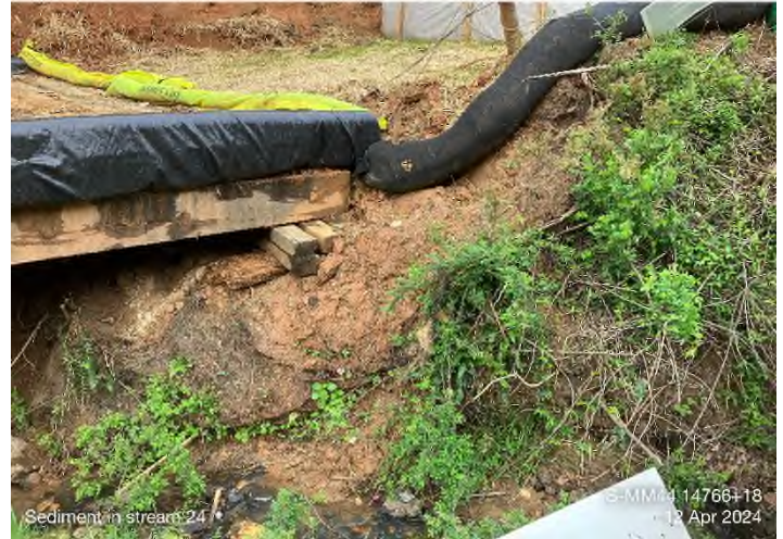
Figure 4: STA 14791+00 – Restabilize fill slope.
