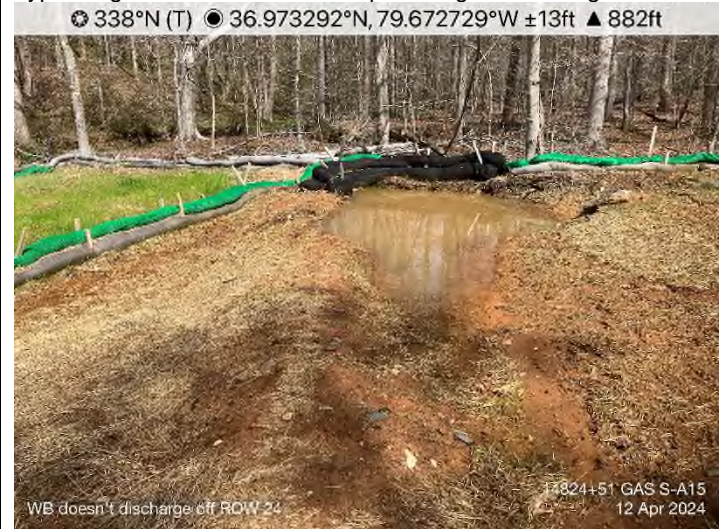
Figure 6: STA 14824+51 – Waterbar is unable to discharge off ROW above Stream S-A15. Outlet is higher than WB causing bypassing endtreatment and compounding WB drainages.
