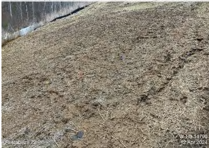
Figure 3: STA 14790+00 – Restabilize and repair rilling above Wetland W-H9.
