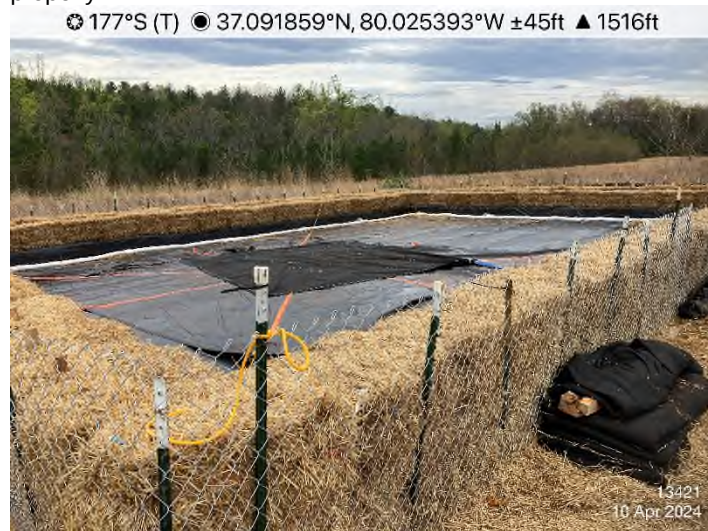
Figure 4: STA 13421+00 – Controls in place and functioning properly.
