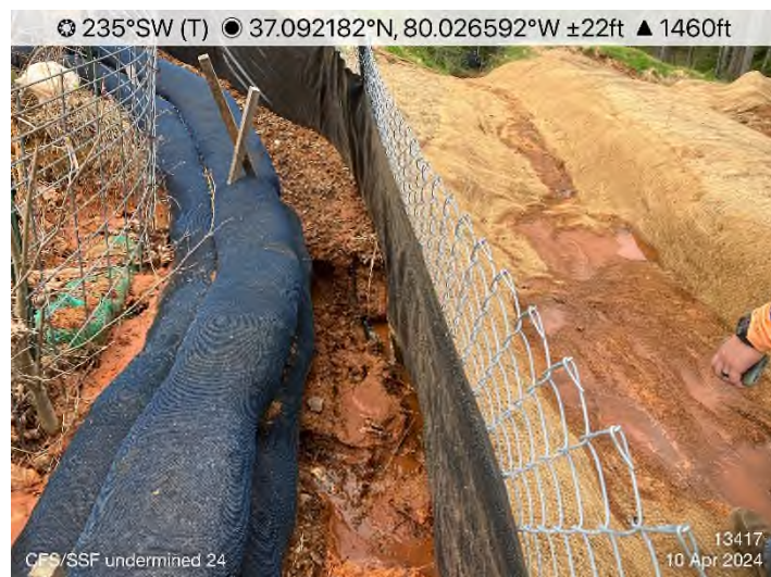
Figure 3: STA 13421+00 – Controls in place and functioning properly.
