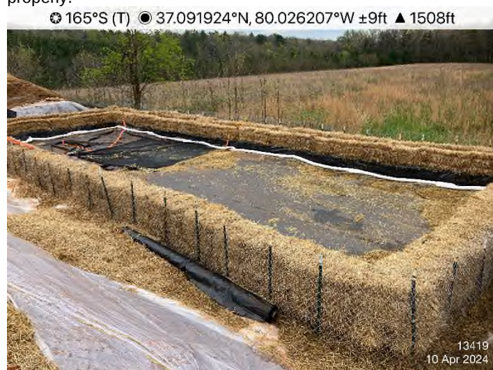
Figure 2: STA 13419+00 – Controls in place and functioning properly.
