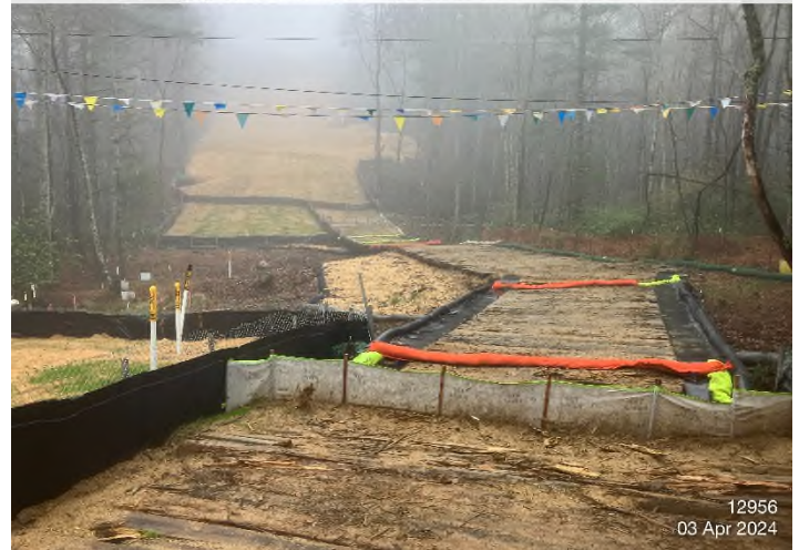
Figure 4: STA 12956+00 – Controls installed and functioning properly.
