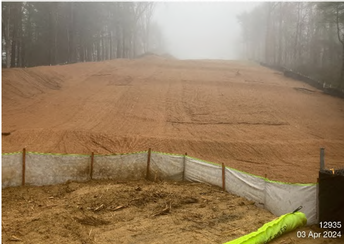
Figure 3: STA 12935+00 – Controls installed and functioning properly.
