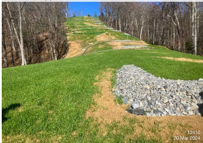
Figure 4: STA 13358+00 – Controls in place and functioning properly.
