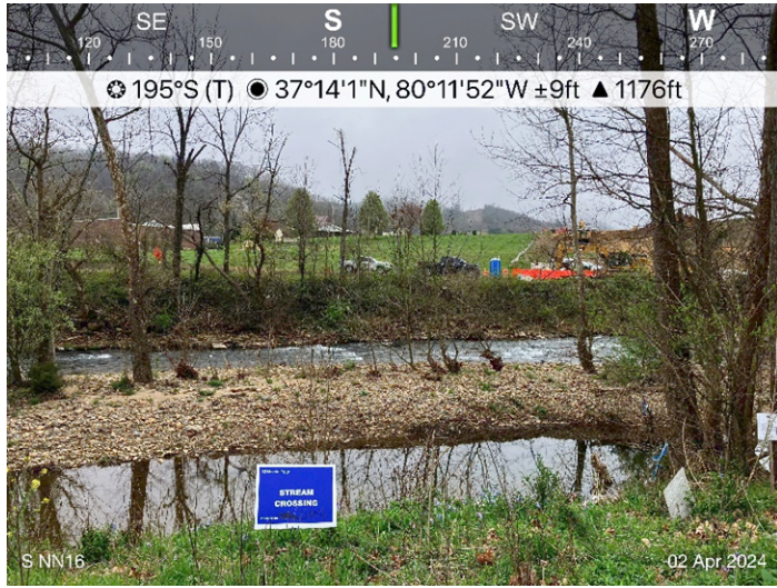
Figure 1: Designated crossing S-NN16, ESC's devices in place.
