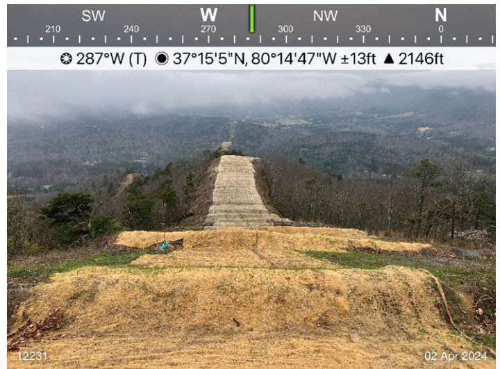
Figure 4: Sta 12231, ESC and stabilization in place.
