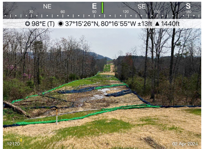
Figure 2: Sta 12120, ESC's devices in place.
