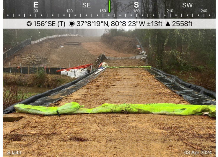
Figure 4: Designated crossing S-IJ43, ESC's devices in place.
