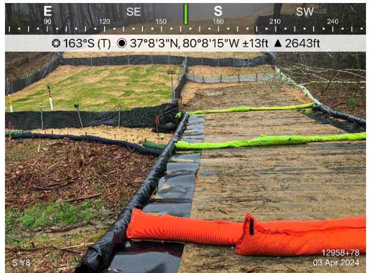
Figure 2: Designated crossing S-Y8, ESC's devices in place.
