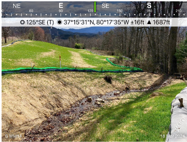
Figure 1: Designated crossing S-MM14, ESC's devices in place.
