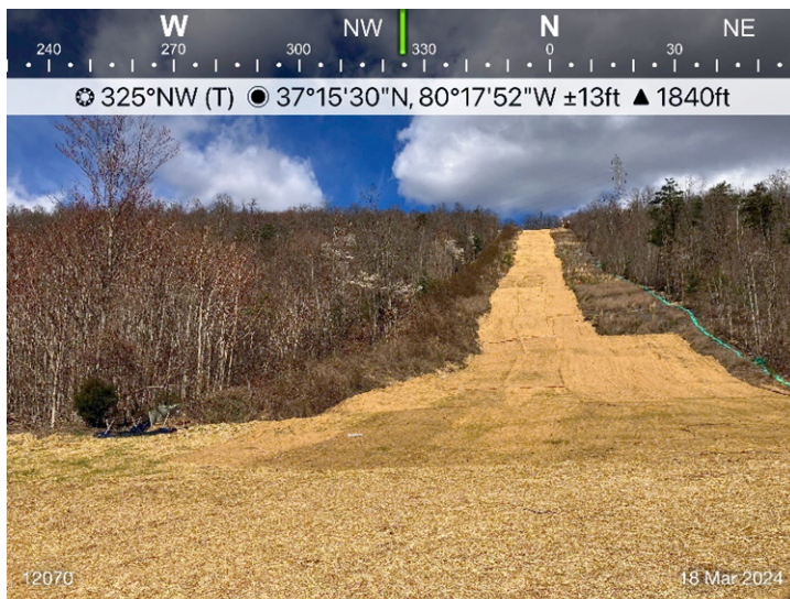
Figure 3: Sta 12070, area is stabilized, and ESC's devices are in place.
