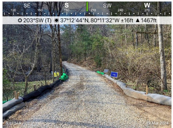
Figure 2: Designated crossing S-EF54A, ESC's devices in place.
