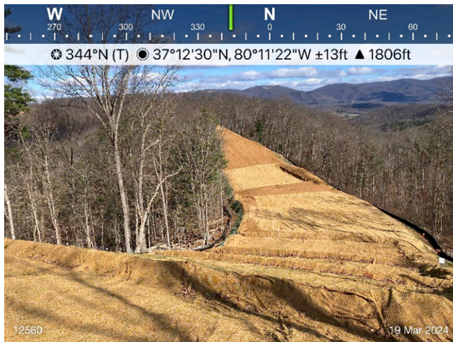
Figure 3: Sta 12560, area is stabilized, and ESC's devices are in place.
