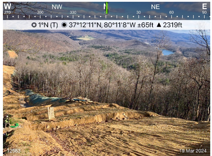
Figure 4: Sta 12583, ESC's devices are in place.
