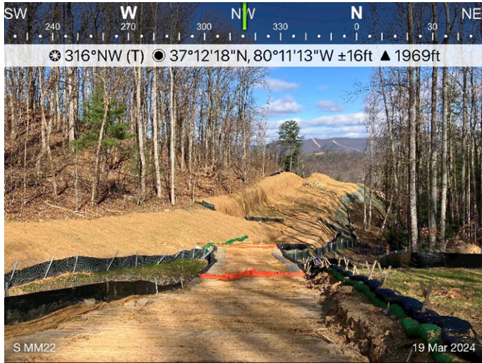
Figure 1: Designated crossing S-MM22, ESC's devices in place.
