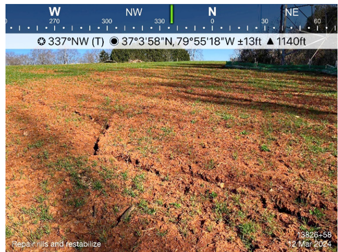
Figure 4: Sta 13826+58 area requires additional stabilization and rill repair.
