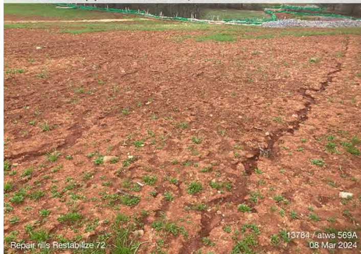
Figure 5: STA 13784+00/ATWS 569A – Repair rills and restabilize denuded areas.
