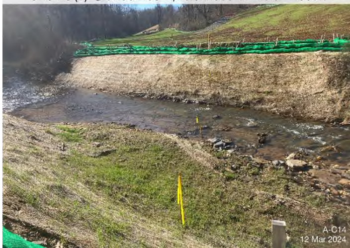
Figure 3: Stream S-C14 – Controls in place and functioning properly.
