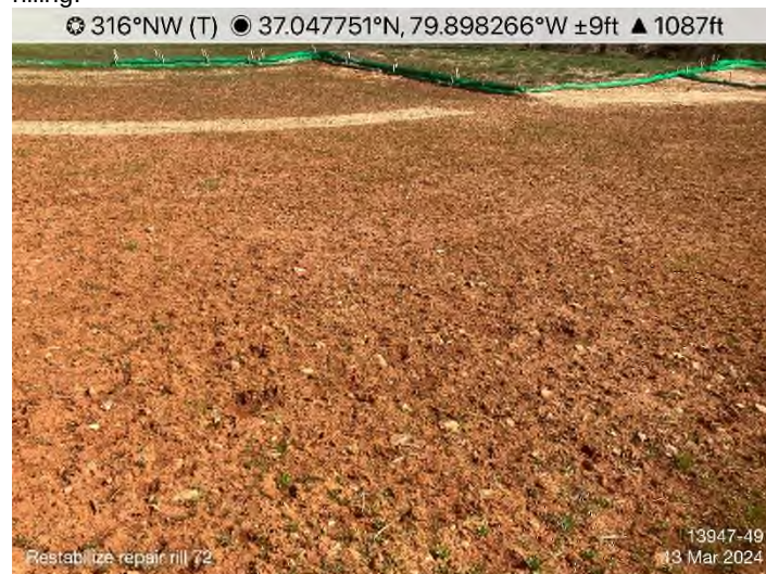
Figure 2: STA 13947+00 to 13949+00 – Restabilize and repair rilling.
