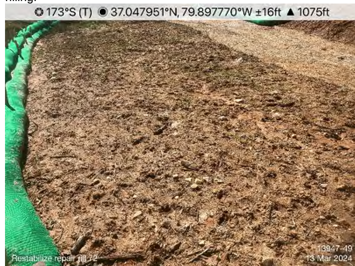
Figure 1: STA 13947+00 to 13949+00 – Restabilize and repair rilling.
