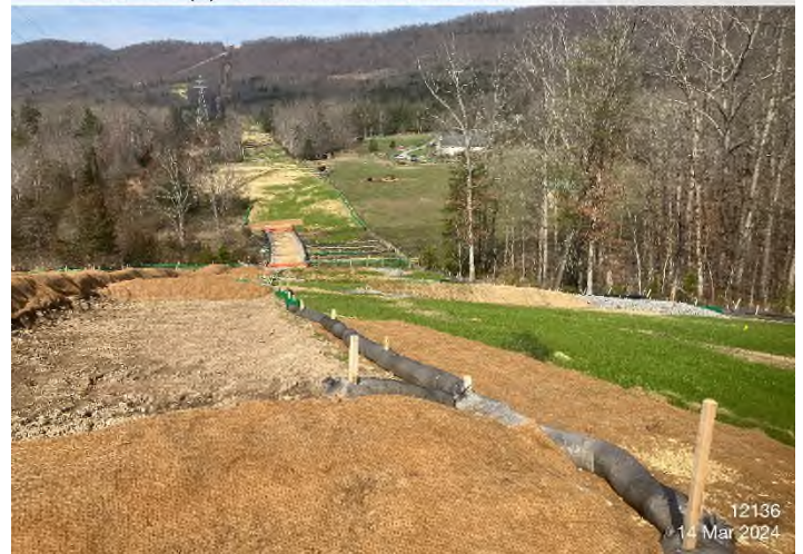
Figure 4: STA 12136+00 – Controls in place and functioning properly.
