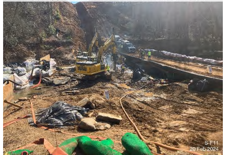
Figure 4: Stream S-F11 – Controls in place and functioning properly.
