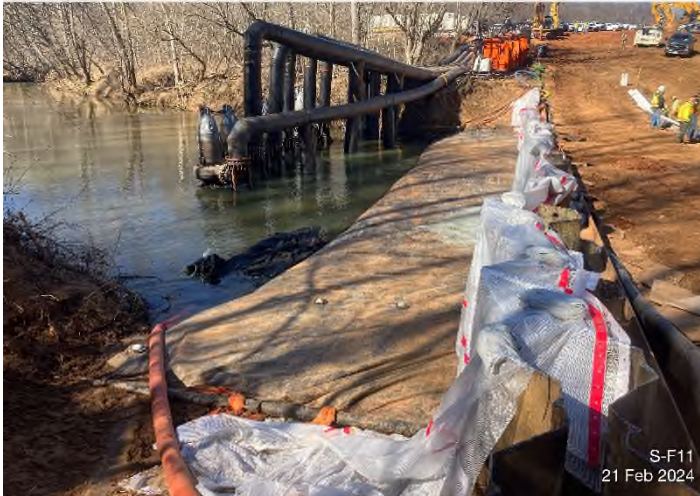
Figure 3: Stream S-F11 – Sediment deposited into the Blackwater River downstream of the ROW crossing. Caused by bank failure due to dewatering operations.
