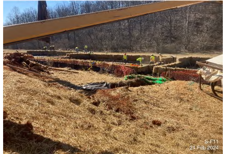
Figure 4: Stream S-F11 – Bank failure down gradient of the dewatering operation.
