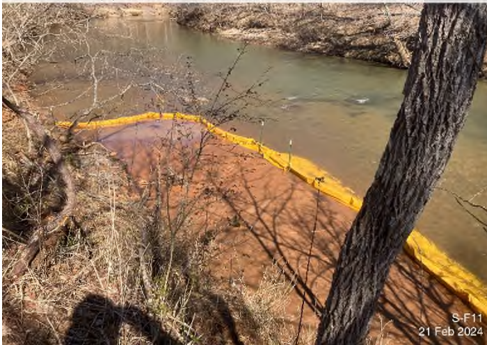
Figure 3: Stream S-F11 – Sediment deposited into the Blackwater River downstream of the ROW crossing. Caused by bank failure due to dewatering operations.
