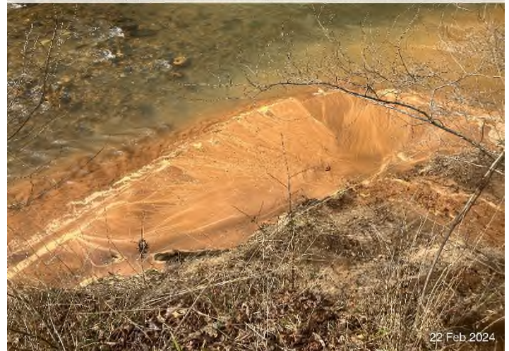
Figure 4: Stream S-C19 – Bank failure down gradient of new dewatering location for S-F11 crossing. Sediment deposited into Magodee Creek.
