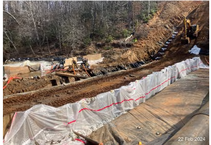
Figure 4: Stream S-C19 – Bank failure down gradient of new dewatering location for S-F11 crossing. Sediment deposited into Magodee Creek.
