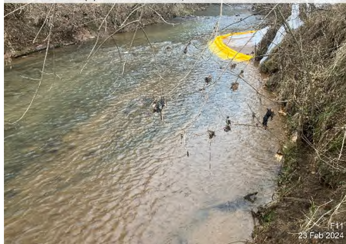
Figure 4: Stream S-C19 – Sediment deposited off ROW from overwhelmed dewatering structures for S-F11.
