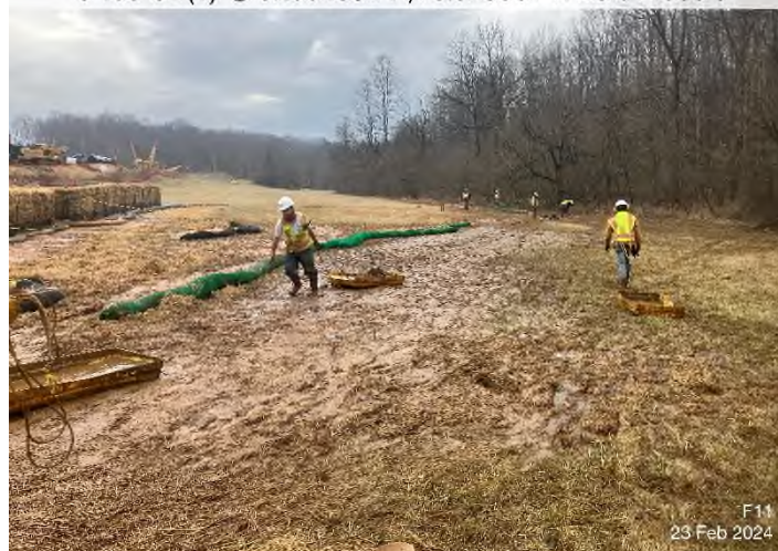
Figure 4: Stream S-C19 – Sediment deposited off ROW from overwhelmed dewatering structures for S-F11.
