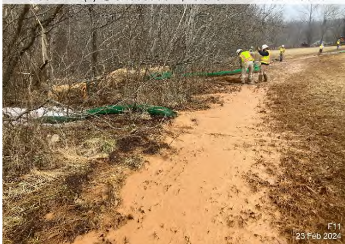
Figure 3: Stream S-C19 – Sediment deposited off ROW from overwhelmed dewatering structures for S-F11.
