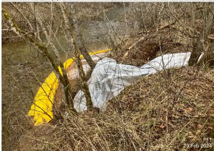
Figure 3: Stream S-C19 – Sediment deposited off ROW from overwhelmed dewatering structures for S-F11.
