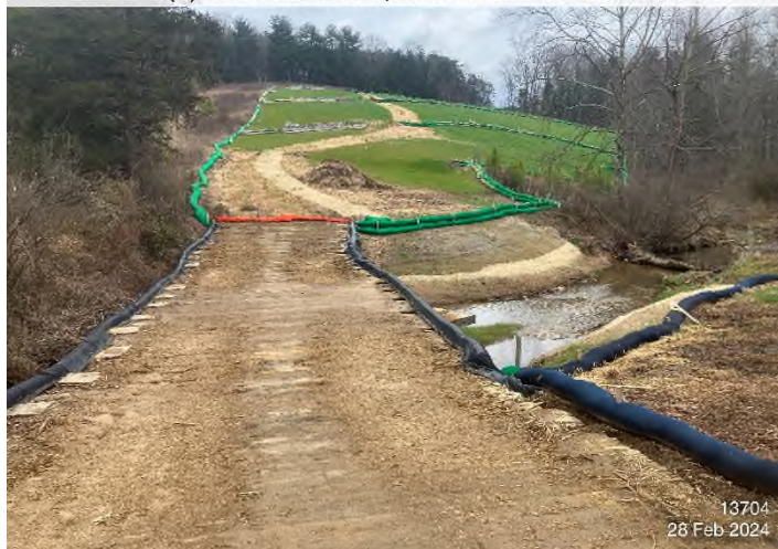
Figure 4: STA 13727+00 – Controls in place and functioning properly.
