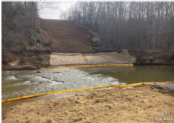
Figure 4: Stream S-F11 – Controls installed and functioning properly.
