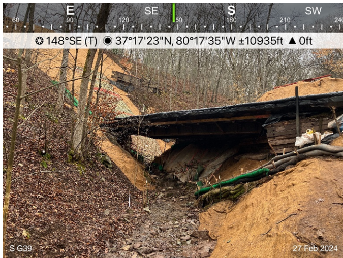
Figure 1: Designated crossing S-G39, ESC's devices in place.
