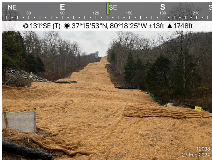
Figure 3: Sta 12038, area is stabilized, and ESC's devices are in place.
