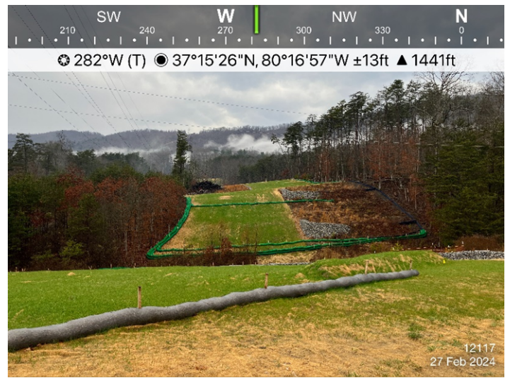
Figure 4: Sta 12117, area is stabilized, and ESC's devices are in place.
