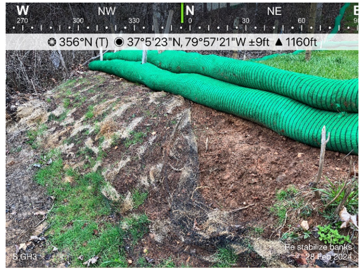
Figure 2: Designated stream S-GH3 banks require re stabilization.
