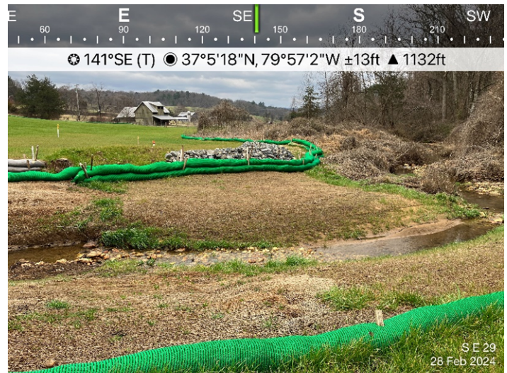
Figure 4: Designated crossing S-E29, ECD's are in place.
