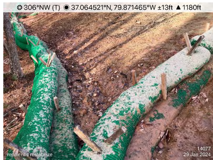
Figure 5: STA 14075+00 to 14077+00 – CFS undermined. Maintenance needed.
