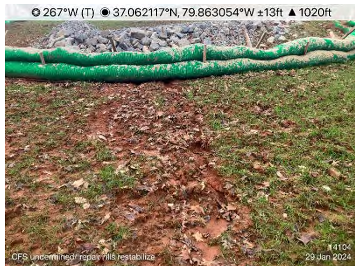
Figure 3: STA 14082+00 to 14083+00 – CFS undermined. Maintenance needed.
