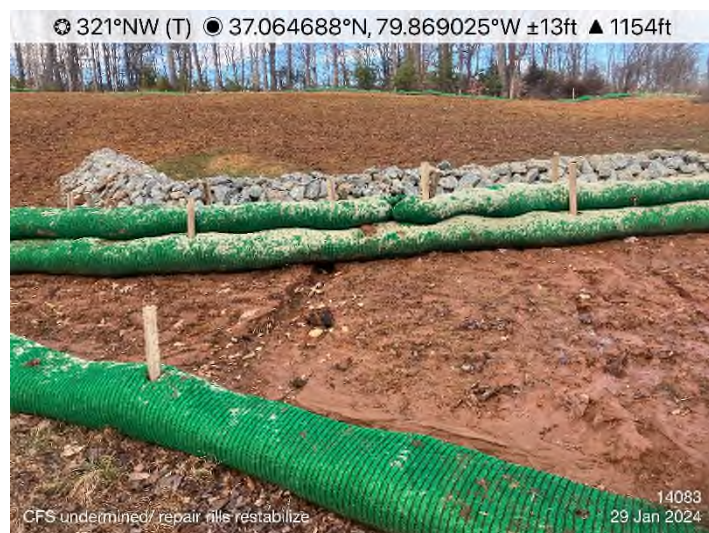
Figure 3: STA 14082+00 to 14083+00 – CFS undermined. Maintenance needed.
