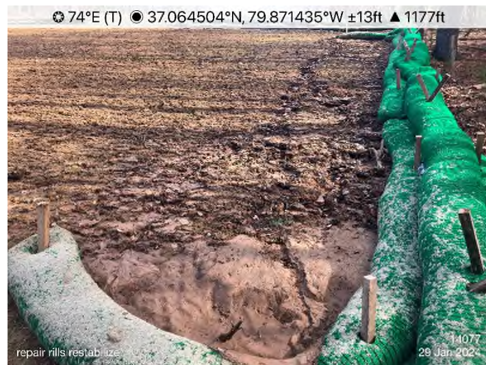
Figure 6: STA 14075+00 to 14077+00 – Repair rilling. Restabilize and reseed as needed.
