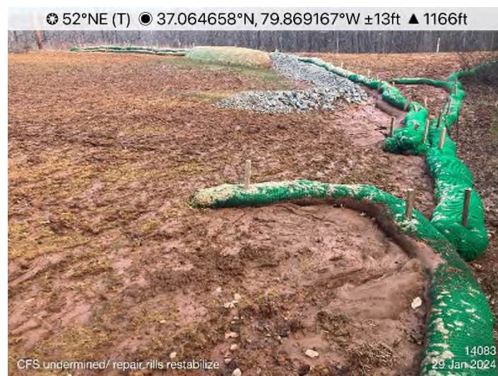
Figure 4: STA 14082+00 to 14083+00 – Repair rilling. Restabilize and reseed as needed.
