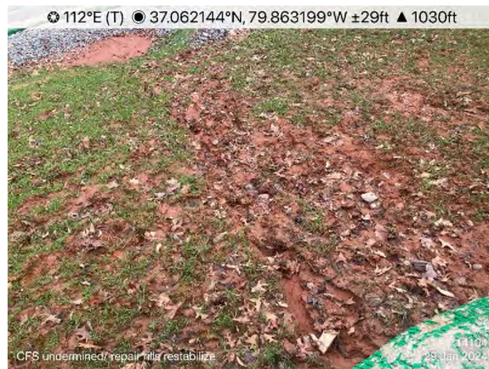
Figure 4: STA 14082+00 to 14083+00 – Repair rilling. Restabilize and reseed as needed.
