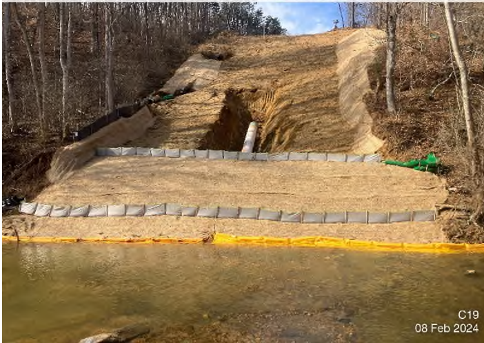
Figure 3: Stream S-C19 – Curlex improperly installed. Edges should be keyed in per the approved details.
