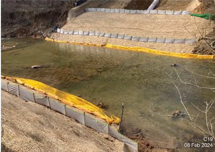
Figure 3: Stream S-C19 – Curlex improperly installed. Edges should be keyed in per the approved details.
