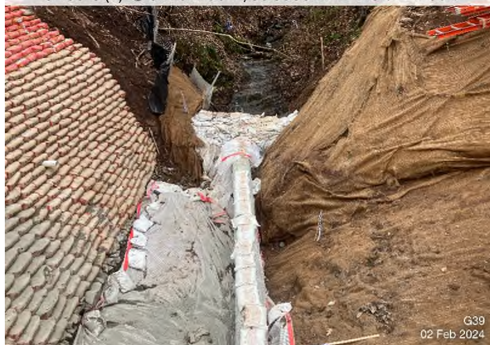
Figure 3: Stream S-EF20a – Controls in place and functioning properly.
