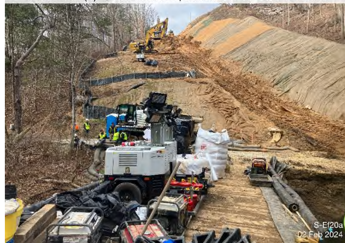
Figure 4: Stream S-EF20a – Controls in place and functioning properly.
