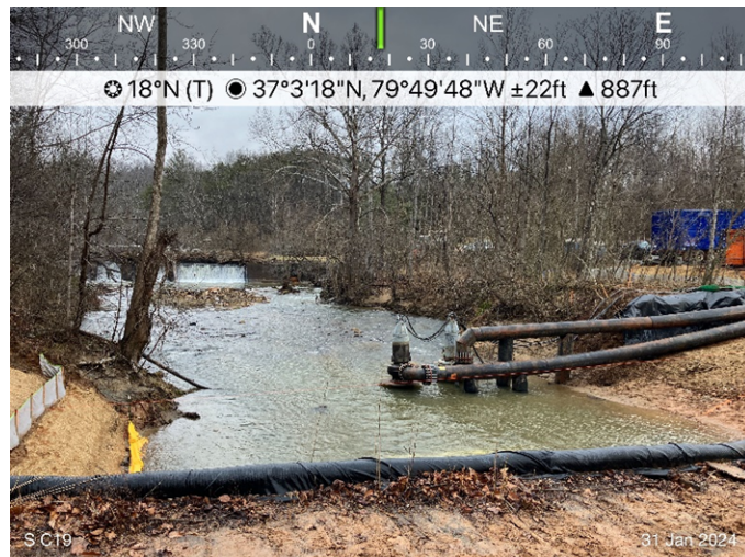
Figure 3: Designated crossing S-C19, ECD's are in place.
