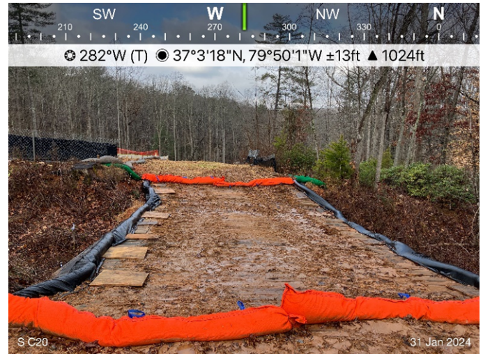
Figure 4: Designated crossing S-C20, ECD's are in place.
