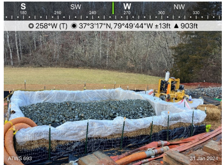
Figure 2: ATWS 693, dewatering structures for S-C19.
