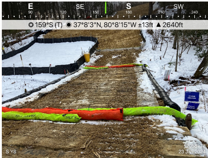
Figure 1: Designated crossing S-Y8, ECD's are in place.
