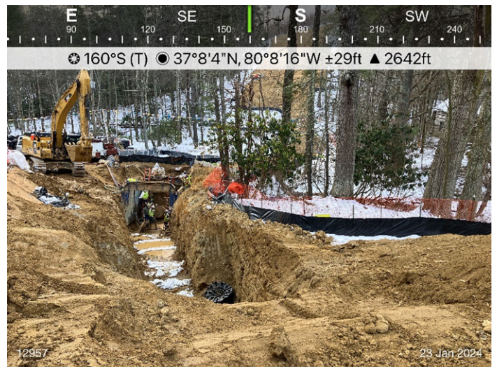
Figure 2: Sta12957, ECD's are in place.
