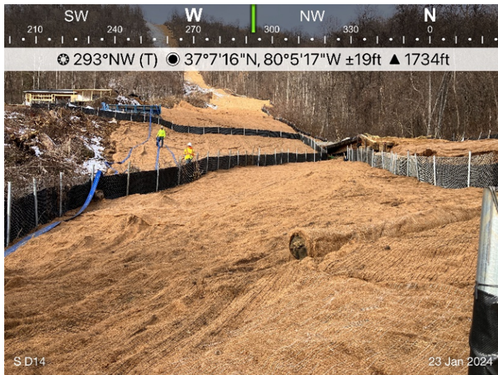
Figure 3: Designated crossing S-D14, ECD's are in place.
