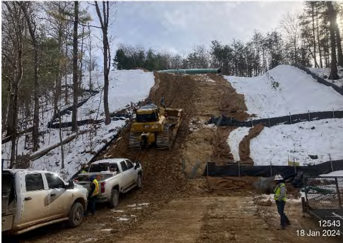
Figure 3: STA 12424+00 – Controls in place and functioning properly.
