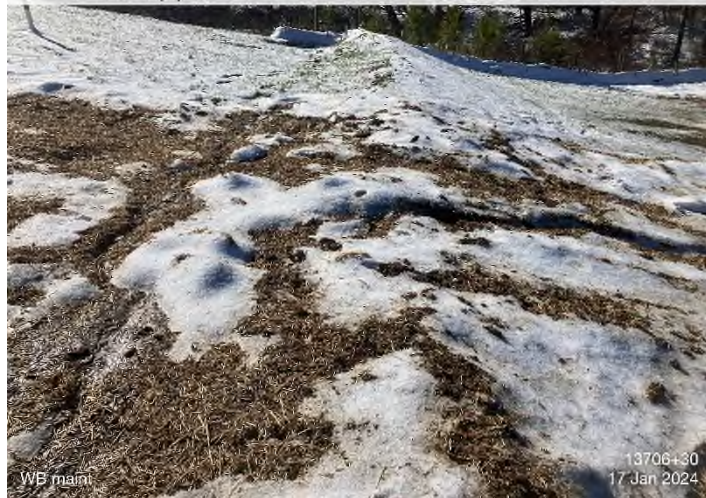
Figure 3: STA 12706+30 – Waterbar topped and needs maintenance.
