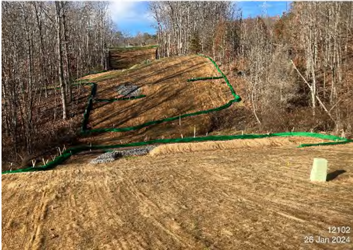
Figure 3: STA 12118+00 – Controls in place and functioning properly.
