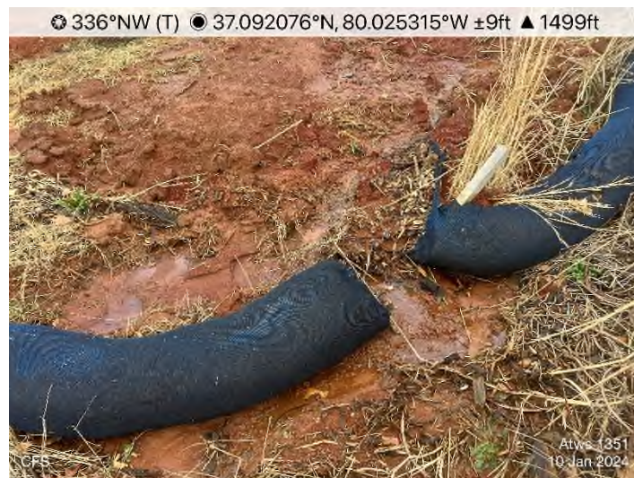
Figure 11: ATWS 1351 – Repair secondary containment.
