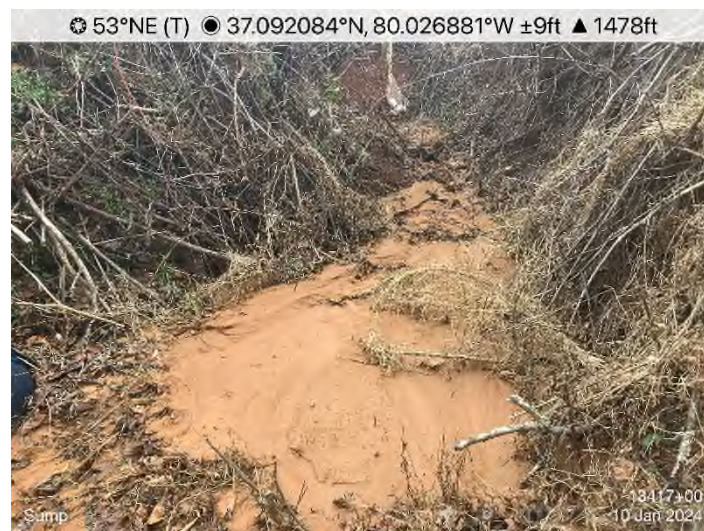
Figure 4: STA 13417+00 – Sump full of sediment.
