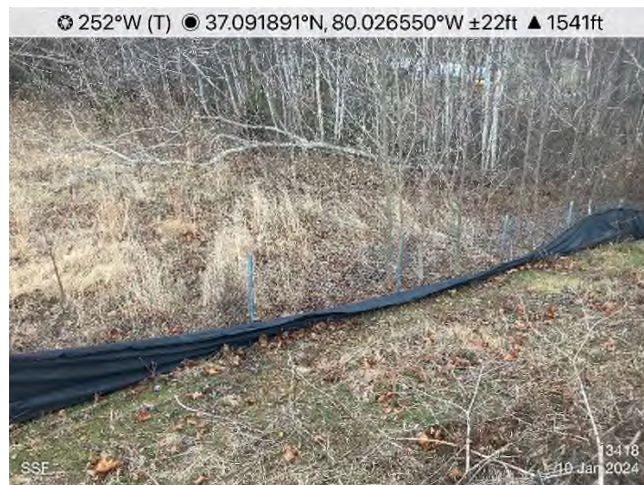
Figure 7: STA 13420+00 – Stabilize stockpiles and fill slopes.
