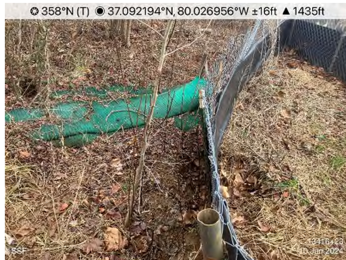
Figure 3: STA 13417+00 – CFS full of sediment.
