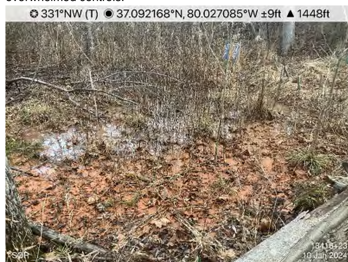
Figure 2: STA 13416+23 – Sediment discharged off ROW due to overwhelmed controls.
