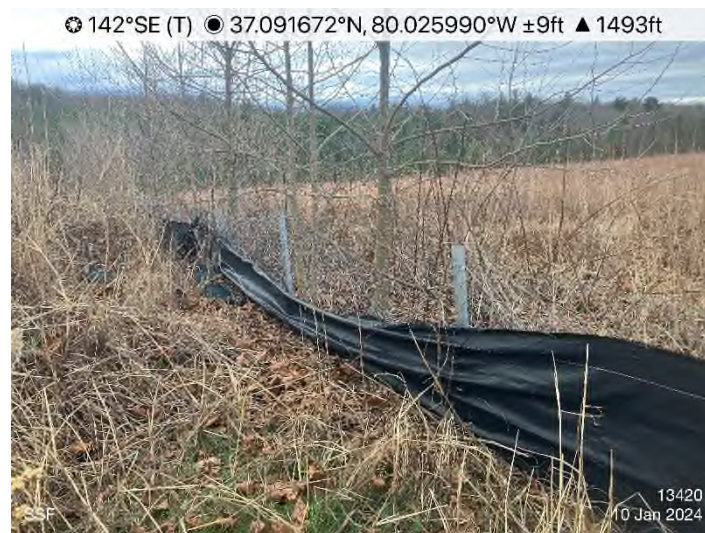
Figure 8: ATWS 1351 – Repair erosion control matting.
