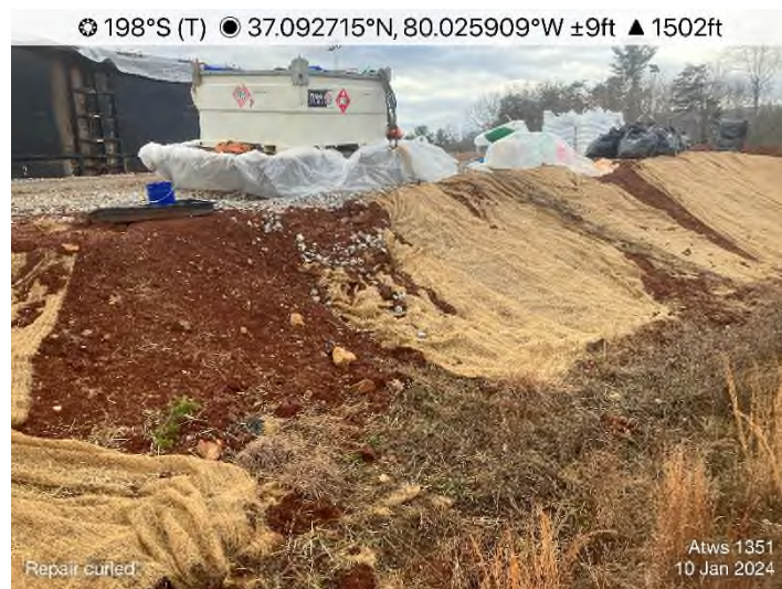
Figure 12: STA 13417+00 – CFS undermined.
