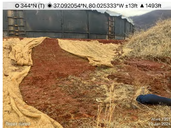
Figure 8: ATWS 1351 – Repair erosion control matting.
