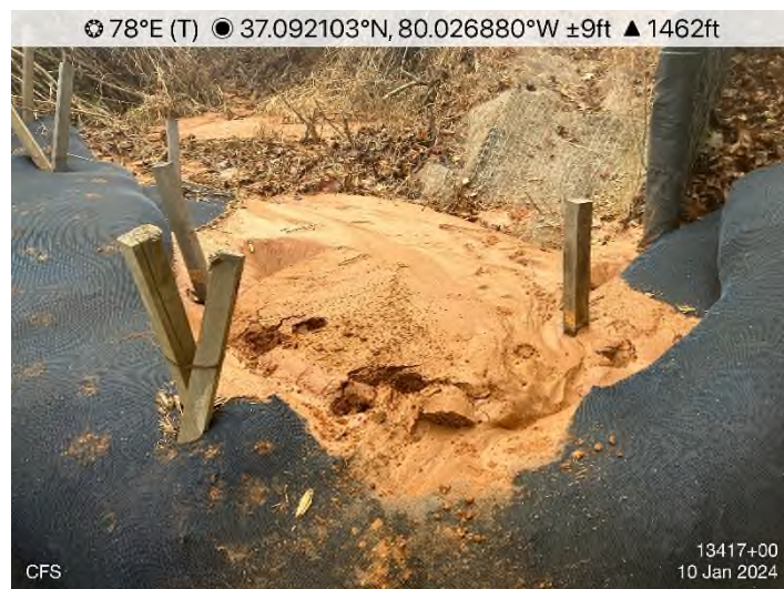
Figure 3: STA 13417+00 – CFS full of sediment.
