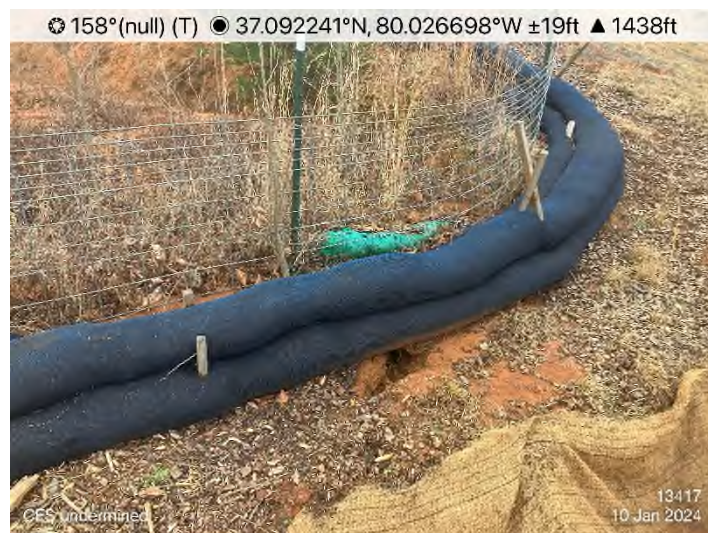
Figure 12: STA 13417+00 – CFS undermined.
