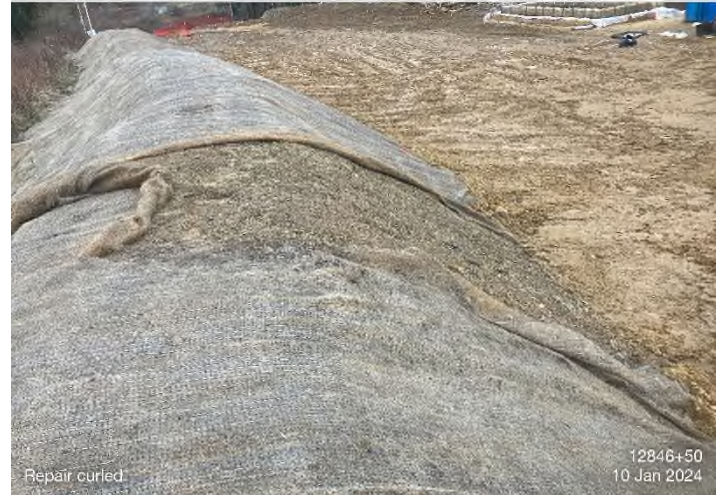
Figure 4: STA 12846+50 – Repair erosion control matting.
