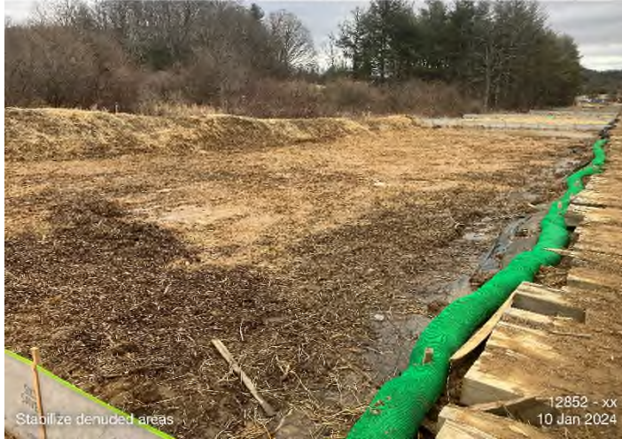
Figure 3: STA 12833+00 to 12865+00 – Seed/stabilize inactive denuded areas.
