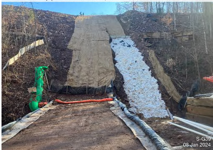
Figure 3: Stream S-G39 – Controls installed and functioning properly.
