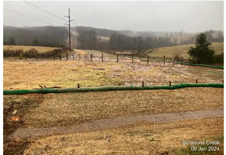
Figure 4: Jacks Creek Road Crossing – Controls installed and functioning properly.
