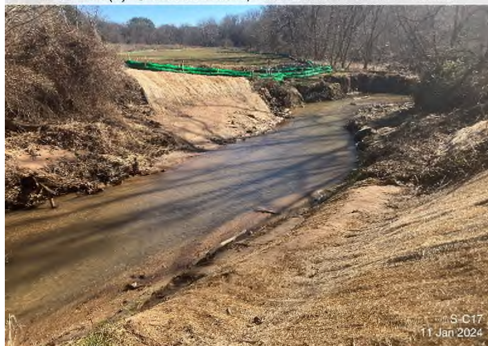
Figure 3: Stream S-C17 – Controls installed and functioning properly.
