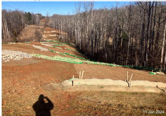
Figure 3: Stream S-C17 – Controls installed and functioning properly.
