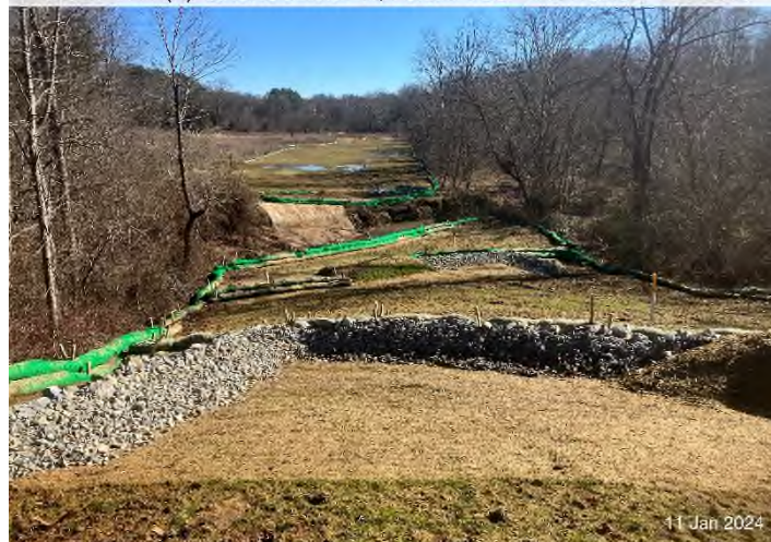
Figure 4: Stream S-CD6 – Controls installed and functioning properly.
