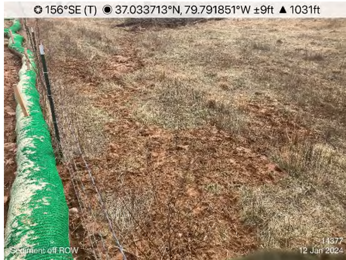
Figure 15: STA 14377+00 – Sediment discharged off ROW from undermined CFS.
