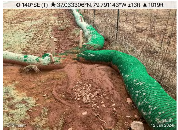
Figure 16: STA 14381+00 – CFS maintenance needed.
