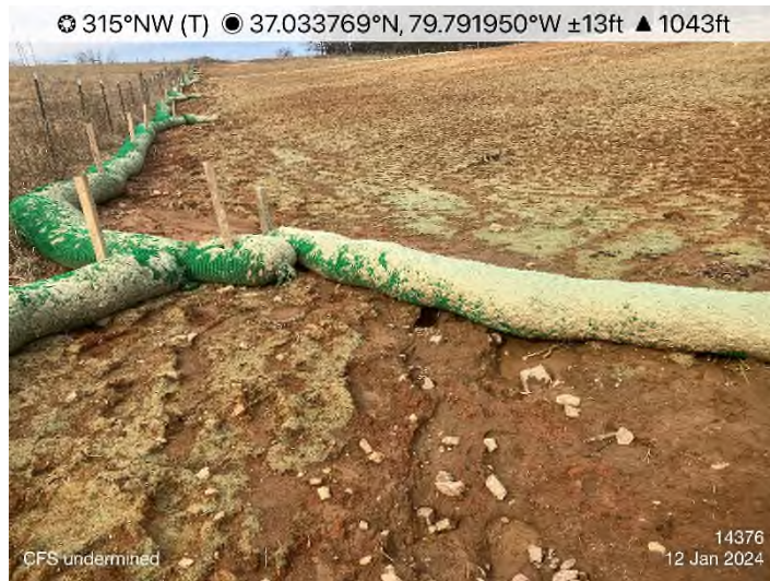
Figure 15: STA 14377+00 – Sediment discharged off ROW from undermined CFS.
