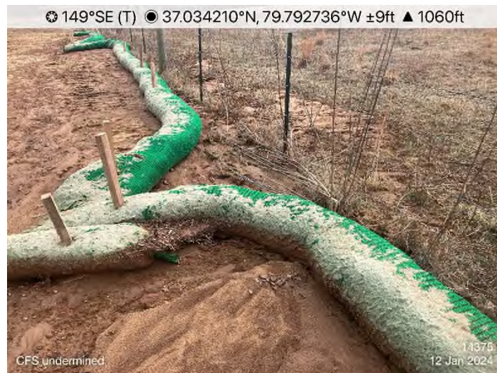
Figure 11: STA 14375+00 – CFS undermined.
