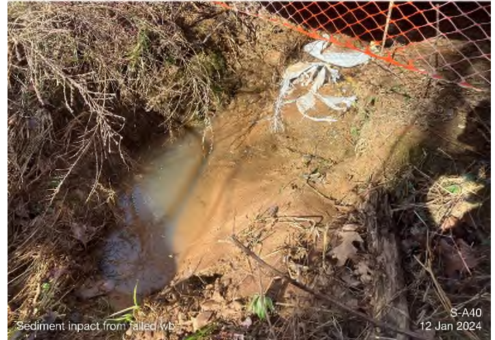
Figure 4: STA 14355+00 – CFS undermined.
