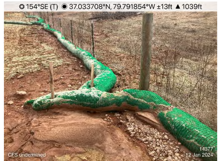
Figure 16: STA 14381+00 – CFS maintenance needed.
