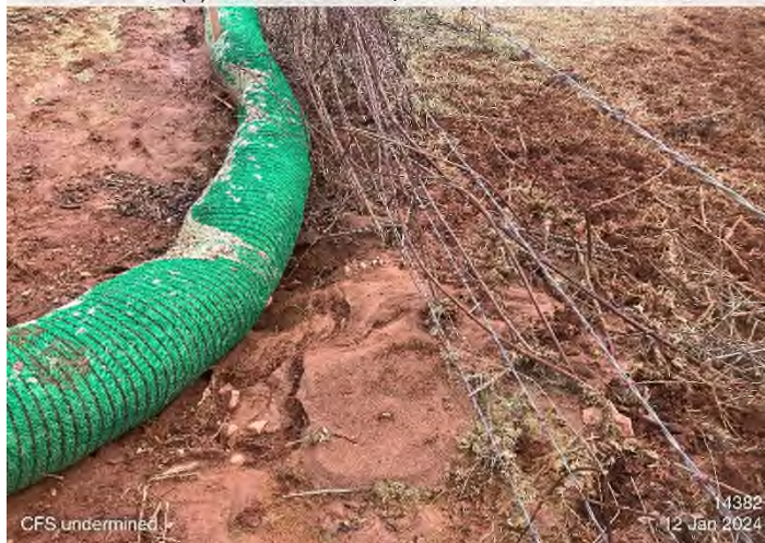
Figure 18: STA 14382+00 – CFS undermined.
