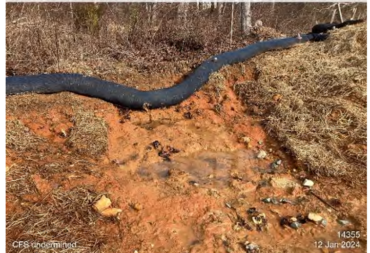
Figure 4: STA 14355+00 – CFS undermined.
