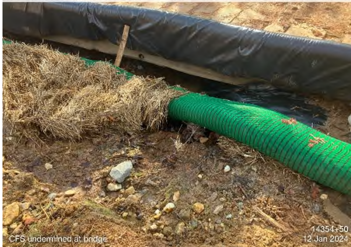
Figure 3: STA 14354+50 – CFS undermined.
