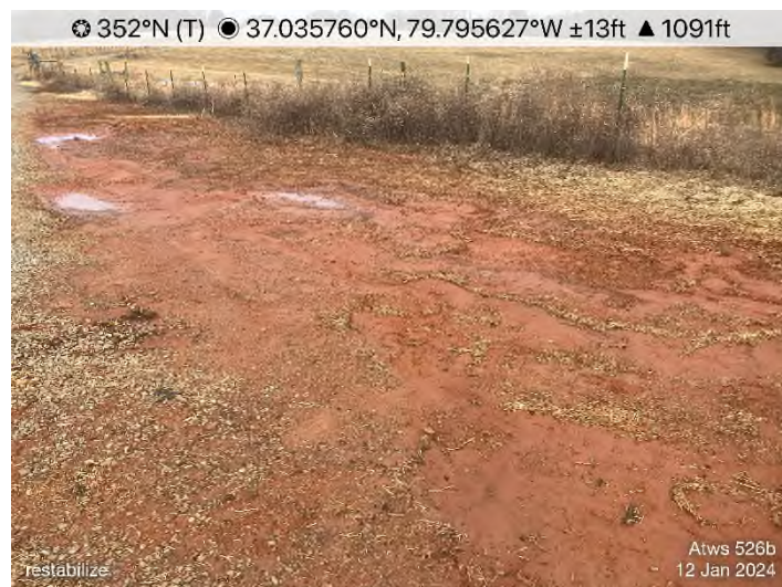
Figure 11: STA 14375+00 – CFS undermined.
