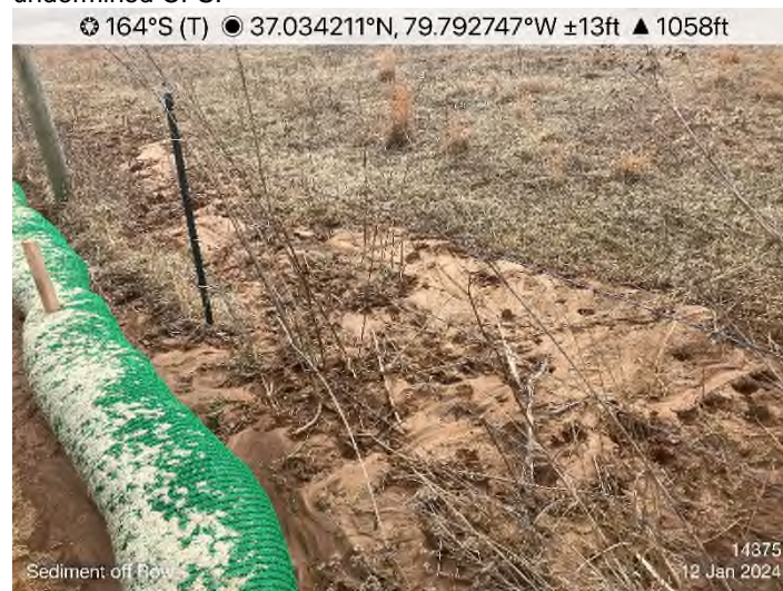
Figure 12: STA 14375+00 – Sediment discharged off ROW from undermined CFS.
